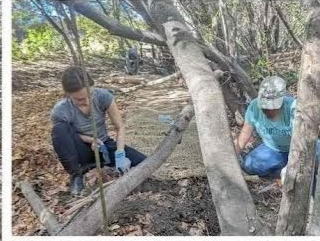
Sept. 30: Installing erosion control at creek edge.
